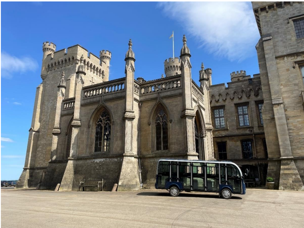
Plate 6: The entrance portico and wider elements of the northwest elevation as seen from west. Note the blocked-in windows on the tower (July 2024).
