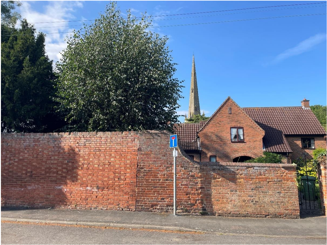
Plate 45: View north towards the Church of St Mary from Church Street, Bottesford (July 2024).
