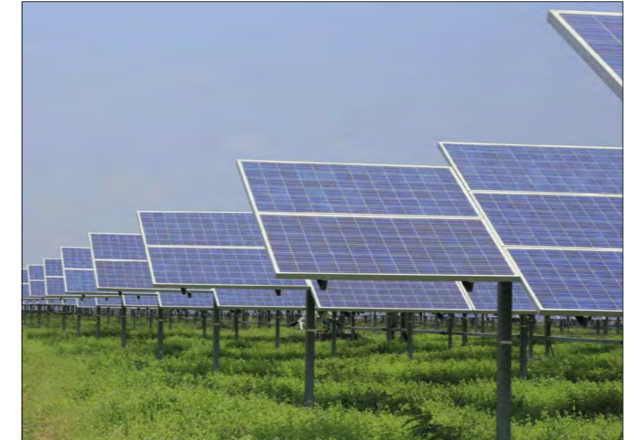
TYPICAL SOLAR PANEL ARRANGEMENT RAISED ABOVE GROUND
