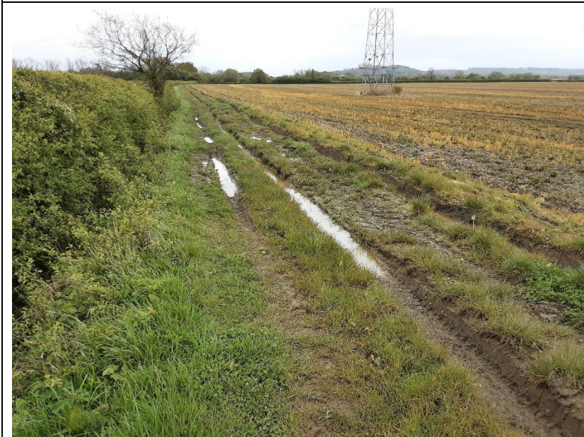
Plate 2: Appeal Site and SSSI boundary (western section, at approximately SK8223671).
