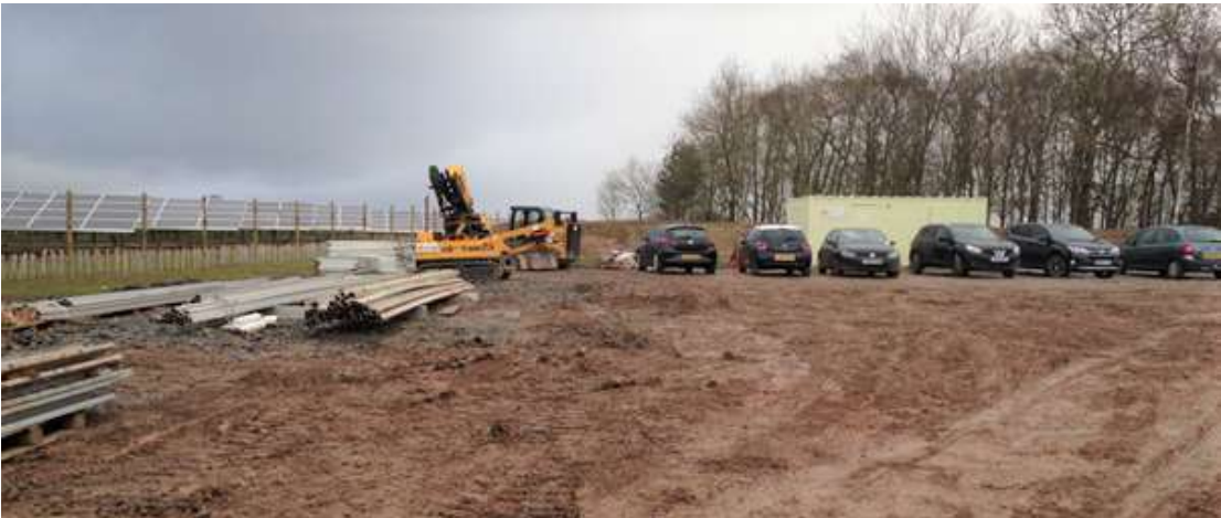
Insert 24: Start of Restoration of Construction Compound
