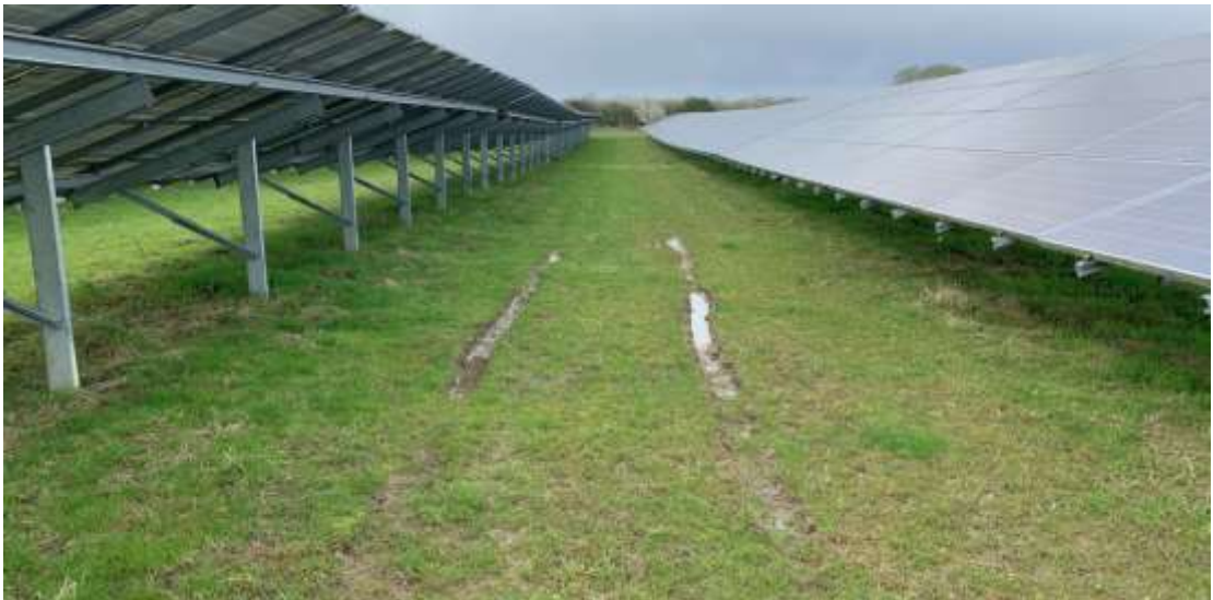
Insert 49: Ruts Caused by Vehicles
