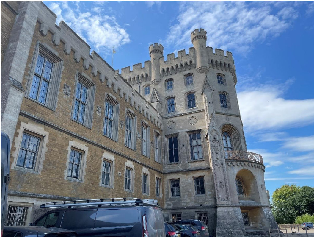
Plate 7.8: Northeast front of Belvoir Castle.
