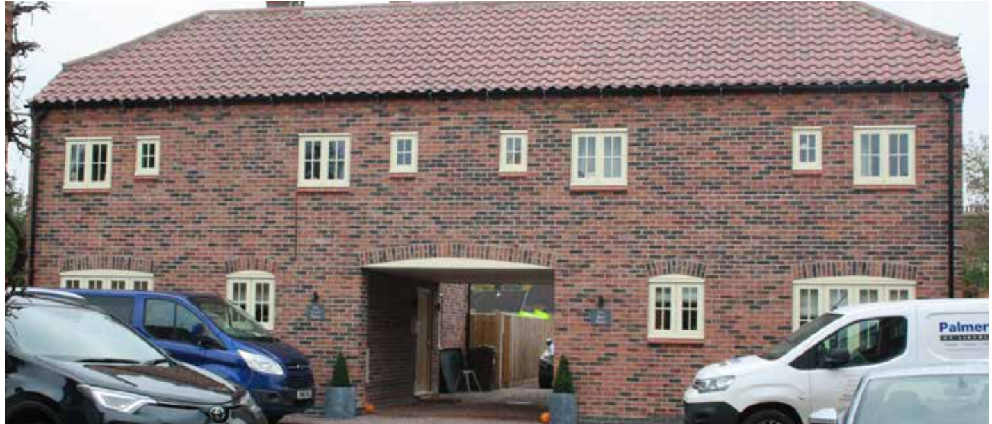
Figure 110: Contemporary homes on Devon Lane red brick façade and clay pantile half hip roof ©Bottesford Parish Council, 2019.
