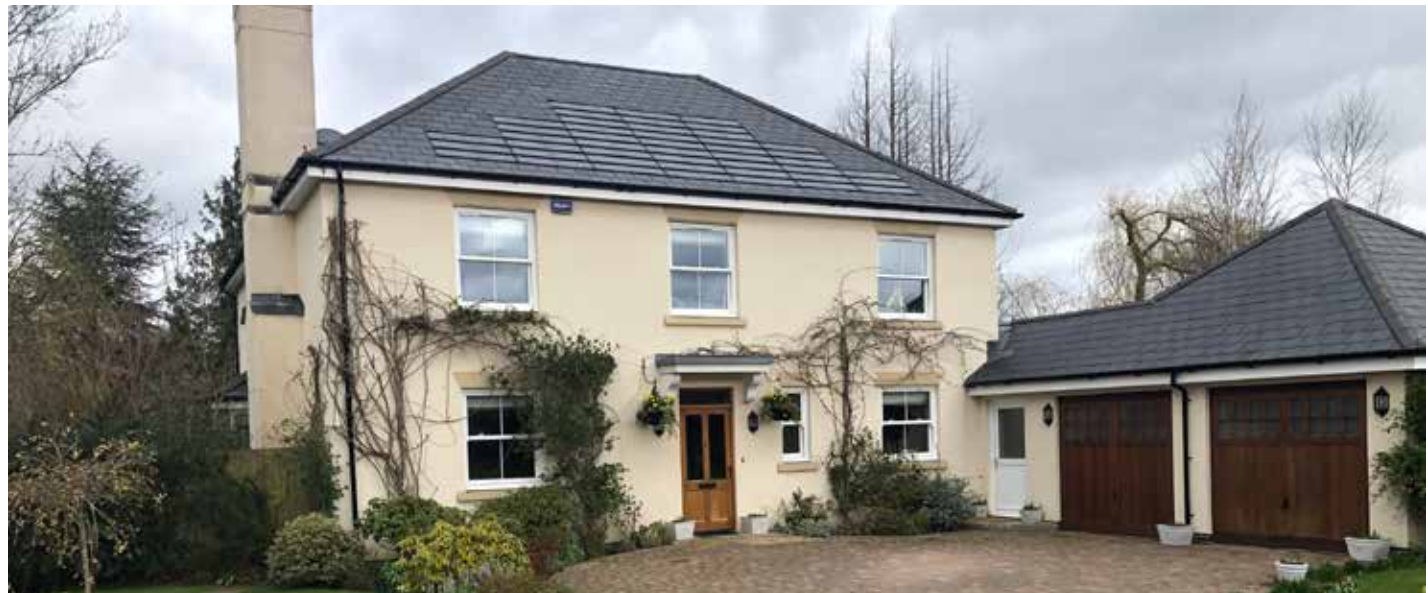
Figure 113: Use of shingle-like solar panels on a slate roof, with the design and colour of the solar panels matching those of the adjacent slate tiles in Lingfield, Surrey.
