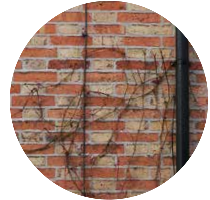
Red and yellow brick laid in Flemish bond
