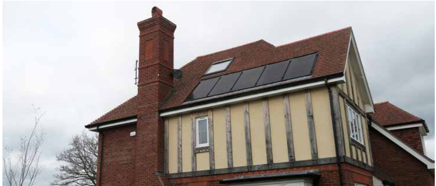
Figure 114: Integration of solar panels on the south-facing pane of the roof of a new house in Lingfield, Surrey.
