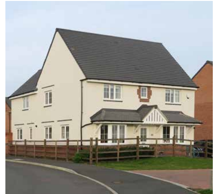
Figure 71: Designs with disproportionate or non-local roofs, bulks, and pitches must be avoided.
