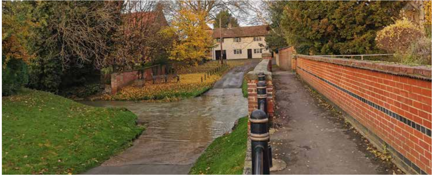
Figure 76: The Grade II-listed footbridge crossing the ford on Devon Lane marks the entrance to the village core. The entrance is highlighted by the singular vehicle crossing of the ford and the green spaces on both sides of the river.
