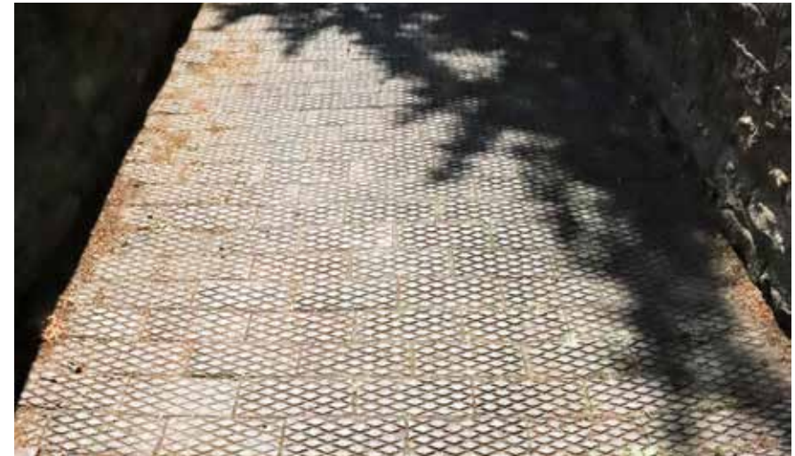
Figure 38: Paving details on Fleming's Bridge ©Bottesford Parish Council, 2020.
