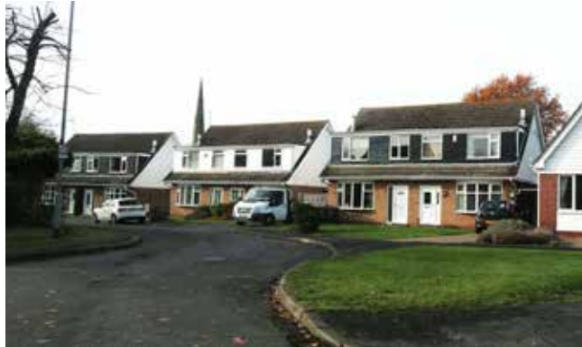
Figure 96: Houses with front garden parking.
