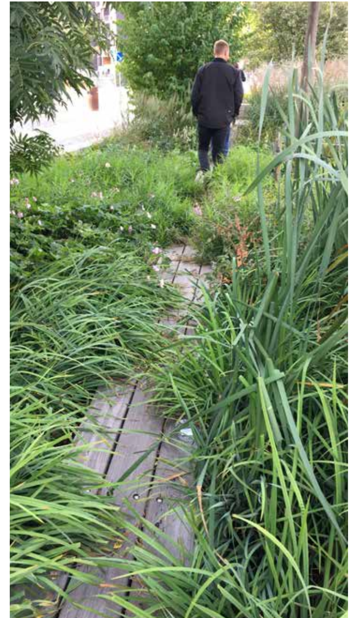
Figure 118: Examples of SuDS designed as a public amenity and fully integrated into the design of the public realm in Stockholm, Sweden.
