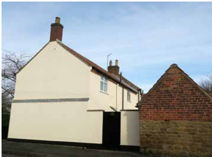
Figure 43: Buildings showing a combination of whitewashed walls (left), red bricks, and ironstone (right), Muston (note: blank walls must be minimised). AECOM
