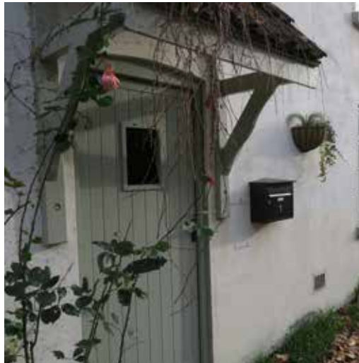
Figure 37: Painted timber door hood, Easthorpe.
