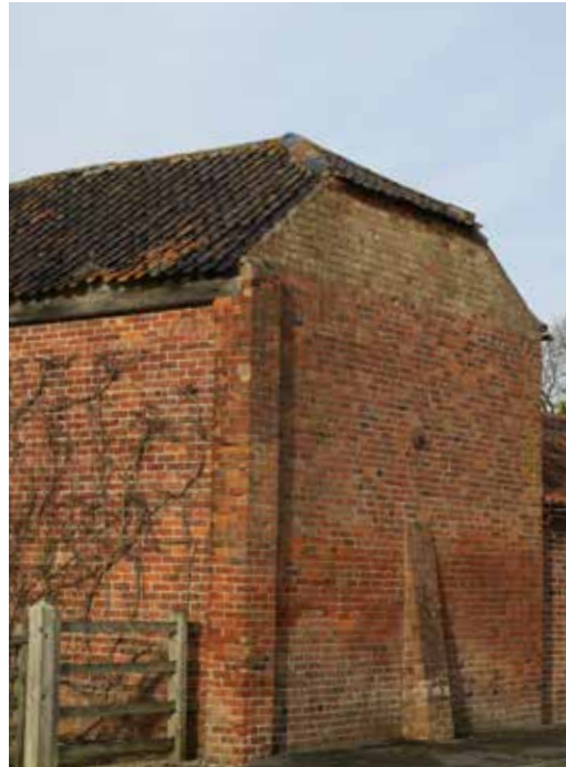
Figure 40: Agricultural building with glazed pantile half hip roof and buttressed red brick wall, Normanton.
