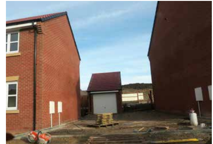
Figure 82: Windows in insufficient number and sizes as well as blank (windowless) walls must be avoided, even on side elevations.
