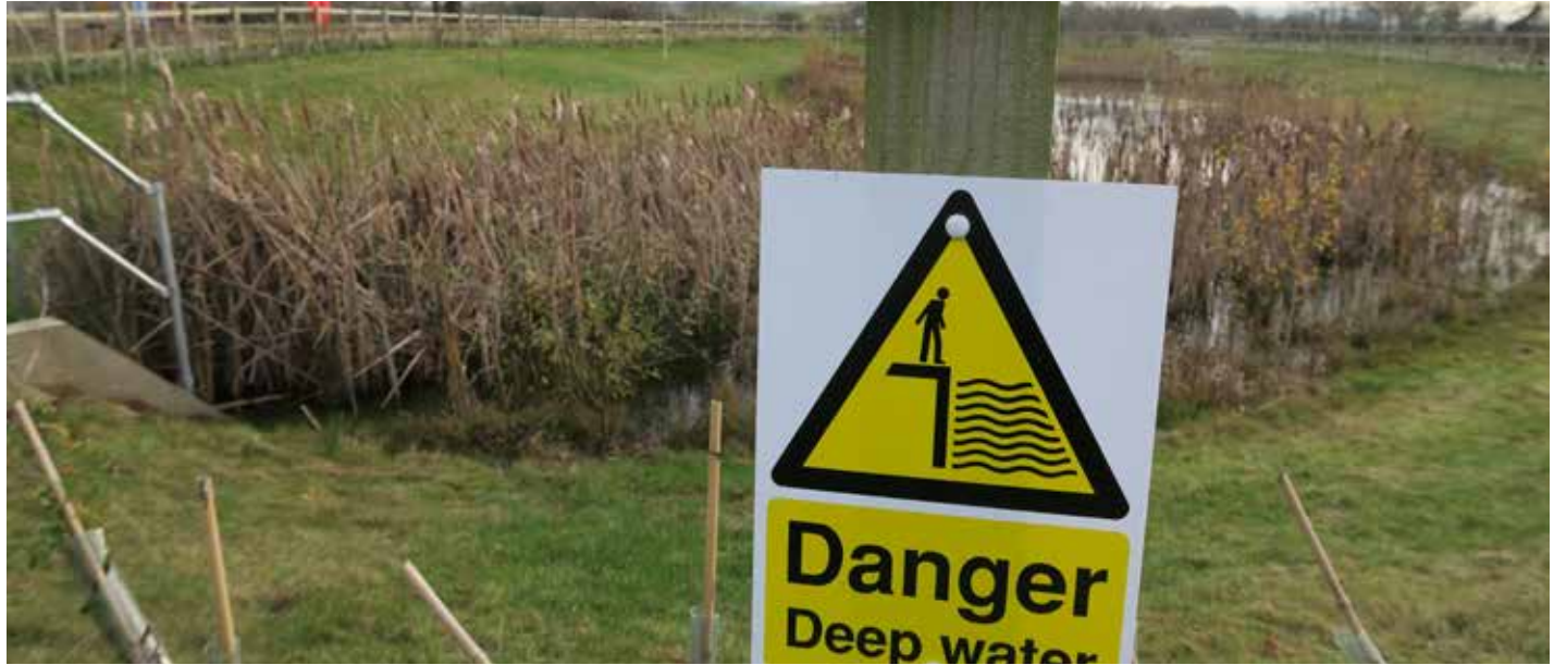
Figure 119: Attenuation ponds and detention basins must be integrated into the green space strategy and designed with safe public access in mind so that they do not necessitate fencing. Designs similar to the facility in Bottesford shown in this picture must be avoided because they are dangerous and have unattractive fencing.
