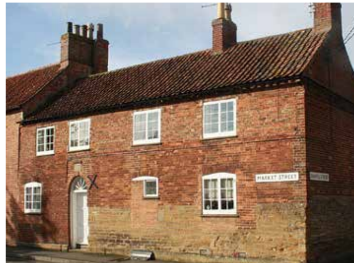
Figure 44: Ironstone and red brick façade, Fleming's Hospital ©Bottesford Parish Council, 2019.
