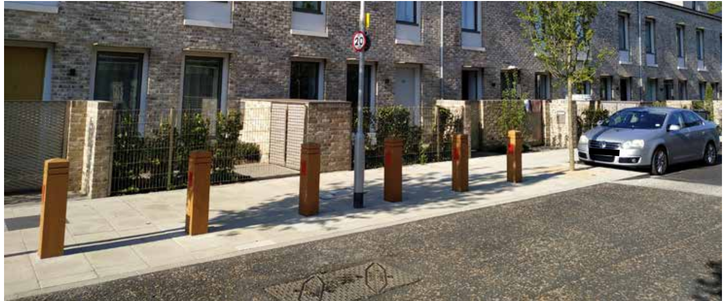
Figure 92: Example of a raised mid-block pedestrian crossing on a 20 mph street on Goldsmith Street, Norwich. (Note: many councils require blister tactile pavers at crossings to guide visually disabled pedestrians and may discourage the use of bollards).
