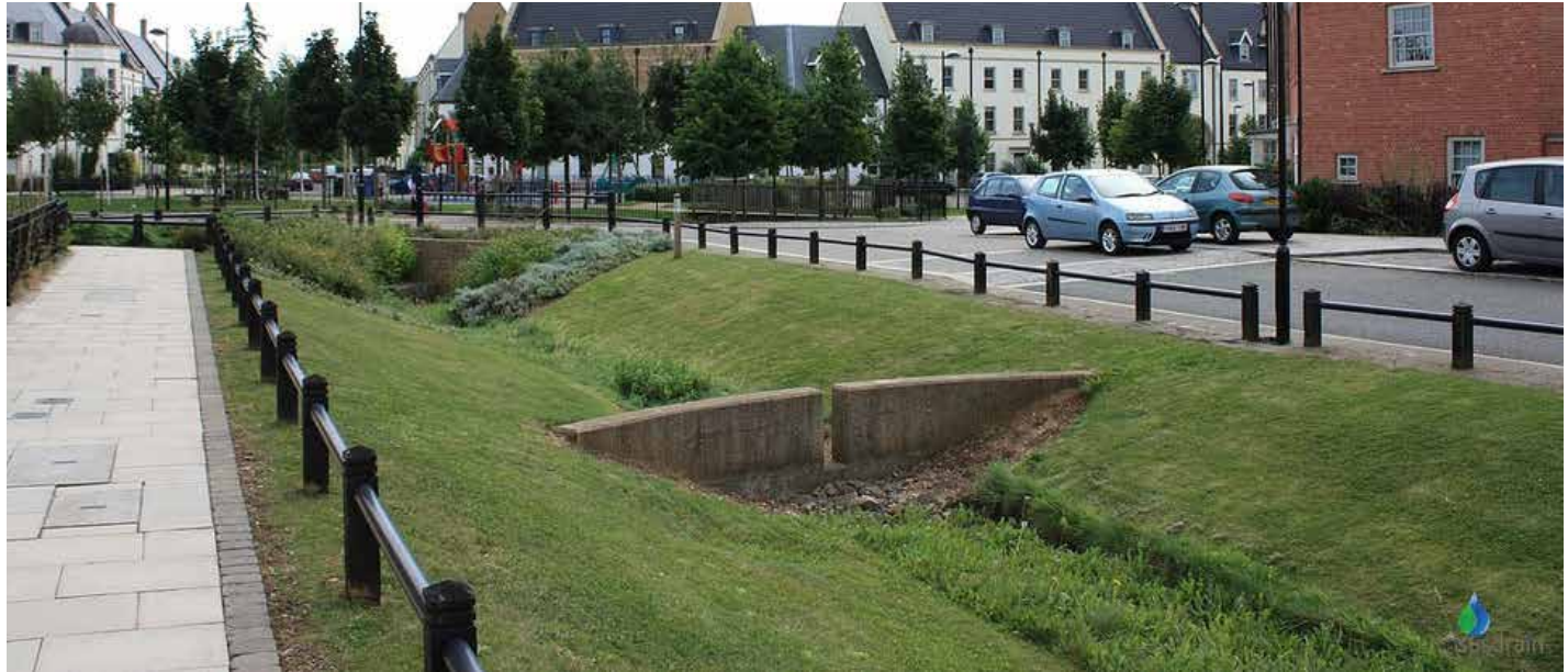
Figure 128: Attenuation swale with check dam (© Susdrain). (Note: the design used in this photo is indicative only; new swales in the Parish must employ context-appropriate designs).
