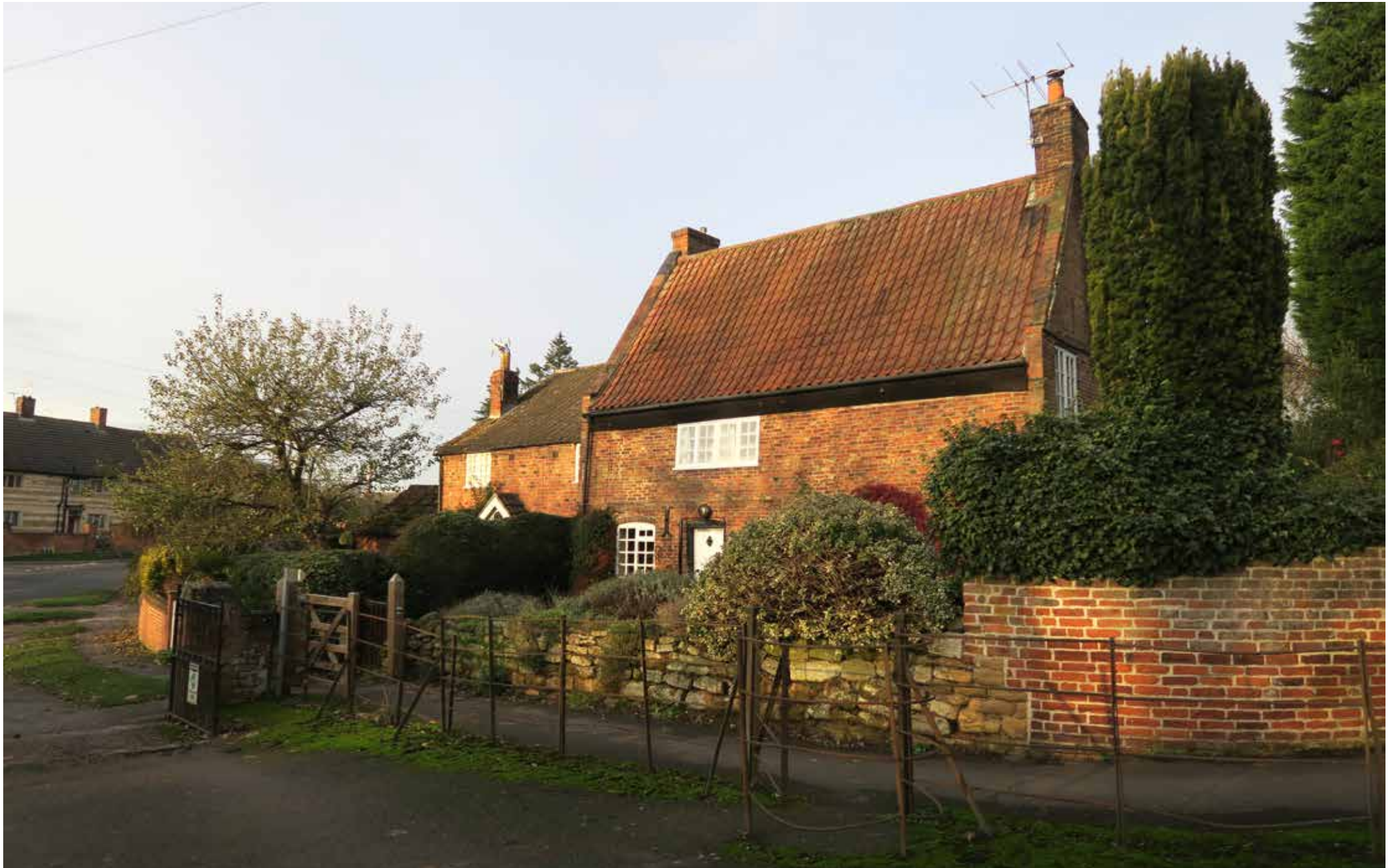
Figure 130: Grade II-listed Providence Cottage.
