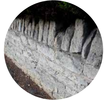
Low stone wall with vertical coping
