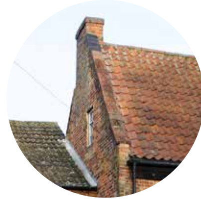
Parapet gable with internal gable-end stacks
