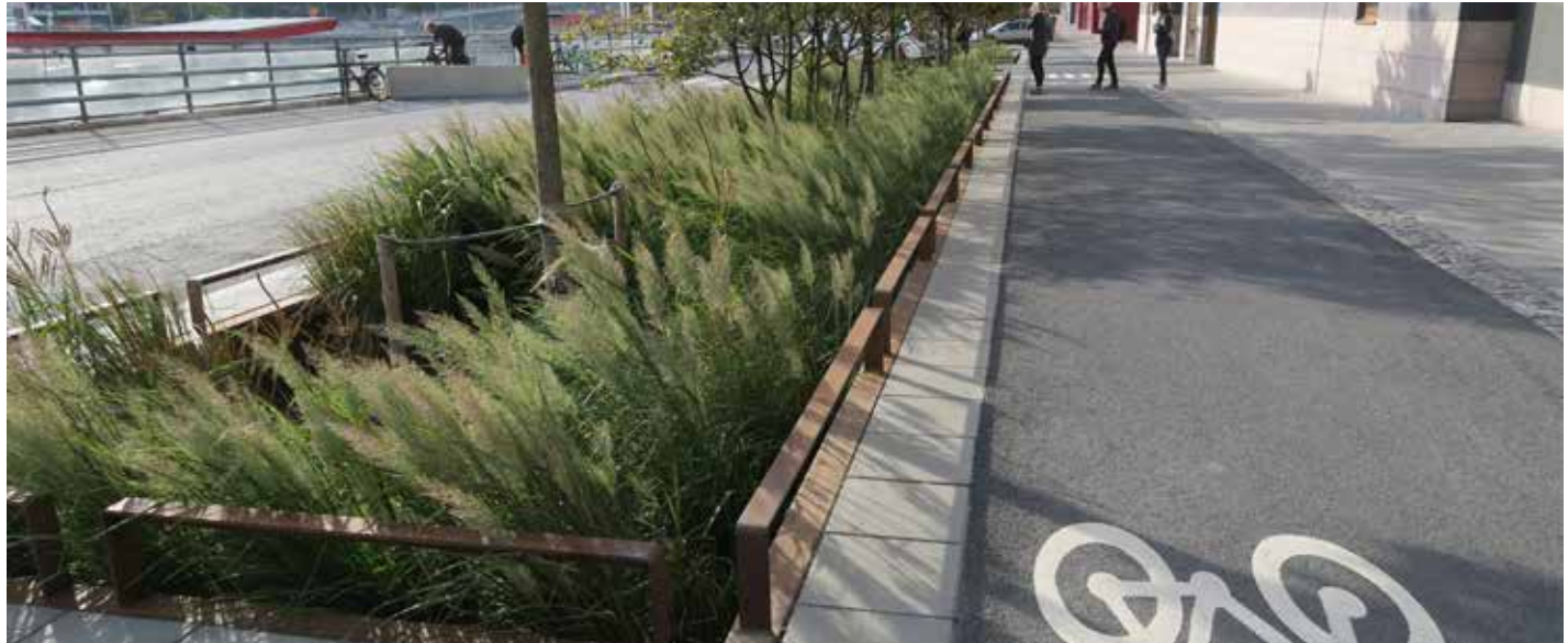
Figure 129: Roadside swale in Stockholm, Sweden. (Note: the design used in this photo is indicative only; new swales in the Parish must employ context-appropriate designs).
