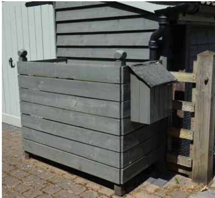
Figure 116: Example of bin storage using the same cladding as the building.
