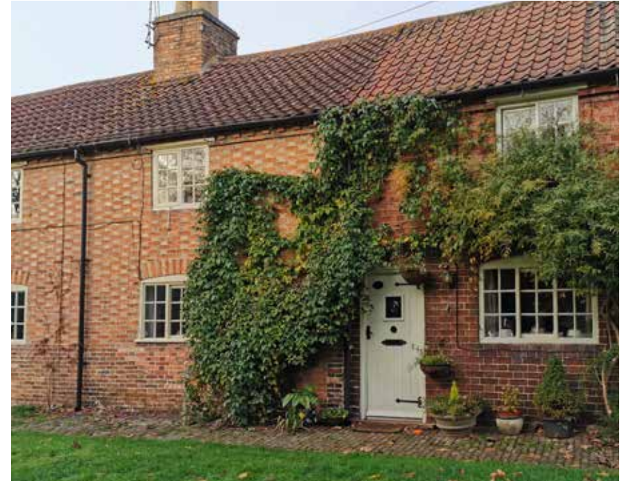
Figure 36: Façade with bicour bricks laid in Flemish bond; ground floor Yorkshire (horizontal) sash window.
