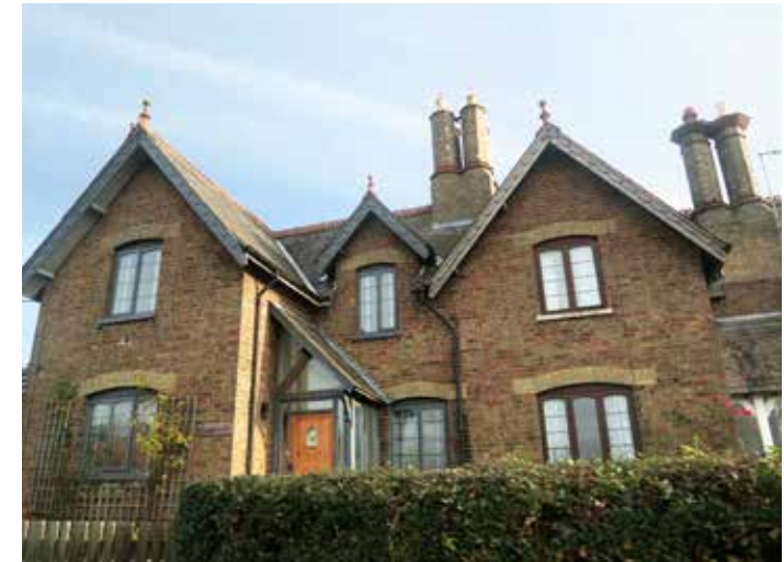
Figure 45: Victorian brown brick house with decorated barge boards, slate roof, and red terracotta ridge and pinnacles, Normanton.
