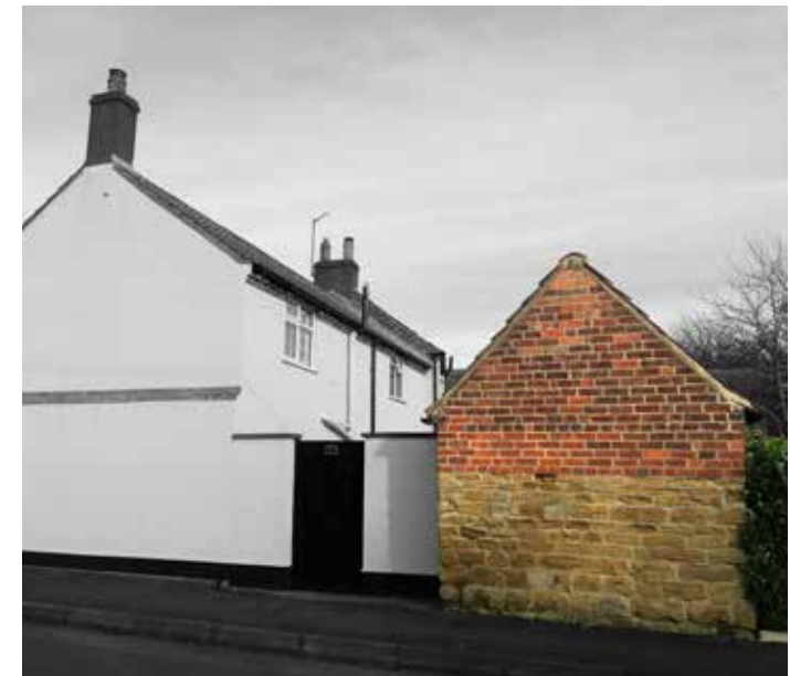
Figure 79: Outbuilding in Muston built in attractive local materials (red brick and ironstone) complementing those of the main building (left).
