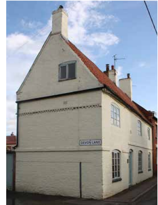
Figure 42: Whitewashed brick gable on Devon Lane and Chapel Street ©Bottesford Parish Council, 2019.
