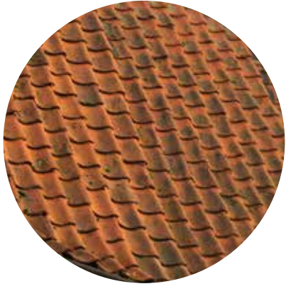
Clay pantile roof
