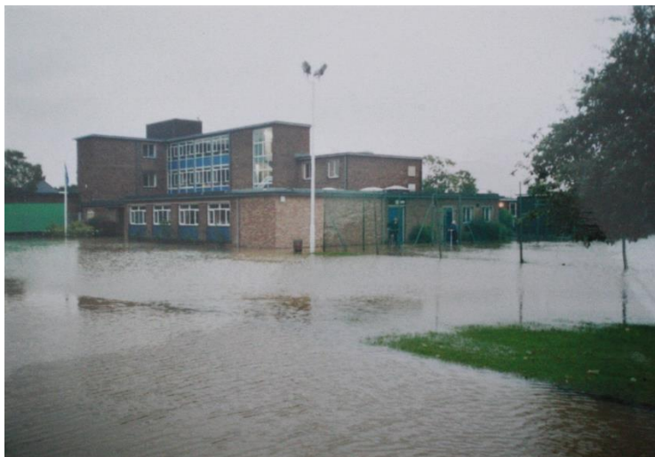
Flooding of the school 2001
