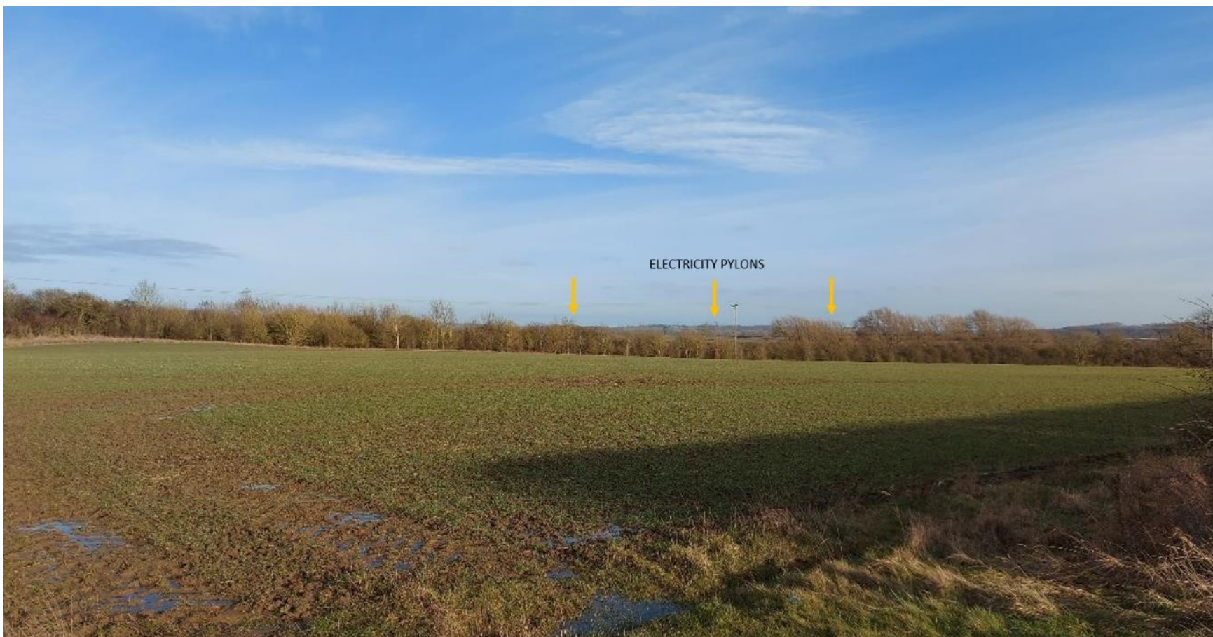
Plate 36: View eastwards towards the site from Toston Hill from break in the hedgerow. The site is beyond the pylons.
