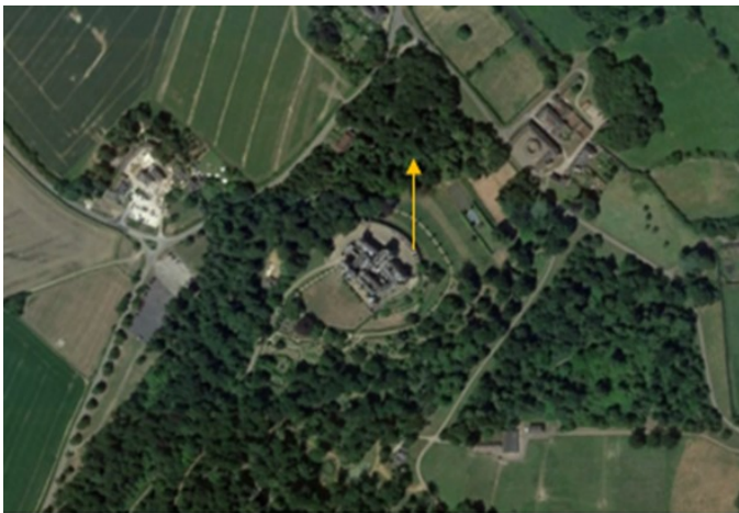
Plate 5: Aerial image of Belvoir Castle showing extensive tree screening to the north of the castle, arrow denotes direction of view of towards the site.
