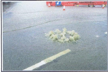
14 th & 15 th June 2016, Main Road at The Sands. Raw sewerage bubbling up into the flood water.
