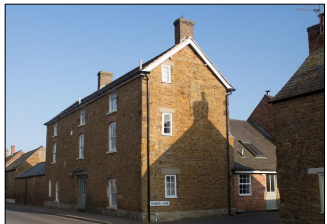
The Bakehouse, early C 18, vernacular dwelling, High Street, Somerby
